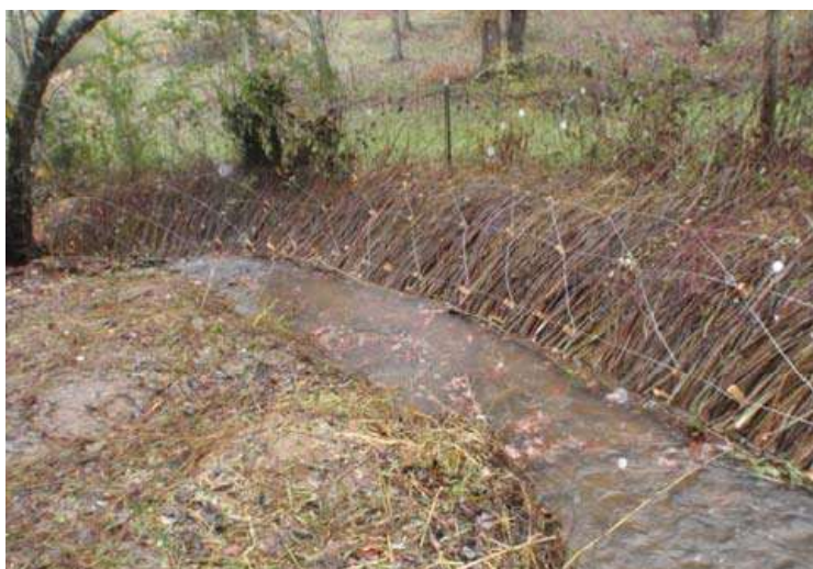
Fig. 1: Installed brush mattress
