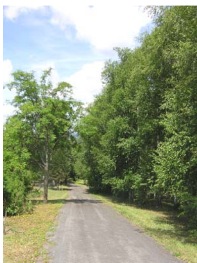
Fig. 3: Example of bituminous roadway
