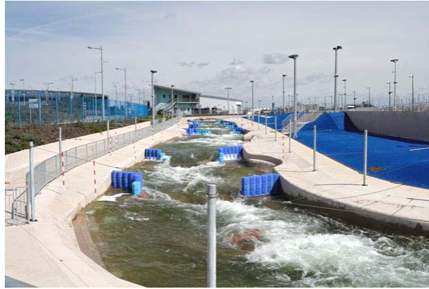
Fig. 1: The Cardiff International Whitewater centre
