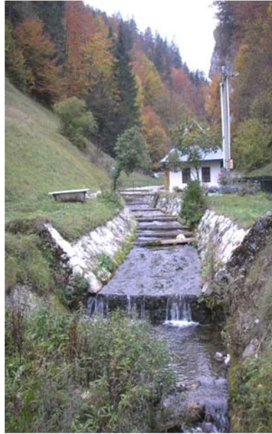
Fig.1 Sills in the torrent control Jelenec
