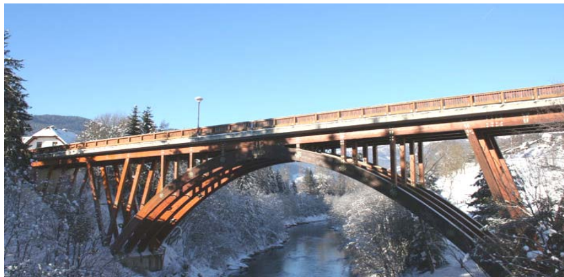
Fig. 1: A pressure treated glulam timber highway bridge in Austria
