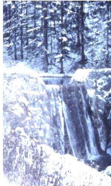
Fig. 2 Dam in the torrent control Jelenec
