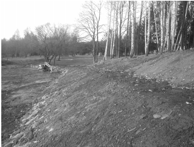
Fig. 5: Bank modification in the area called Sokolské koupaliště, Brno Reservoir [8] [9]
